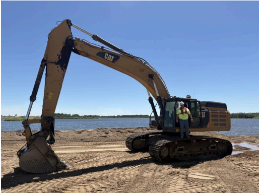
Pictured above: James Haneklaus stands on the new CAT 349 excavator
