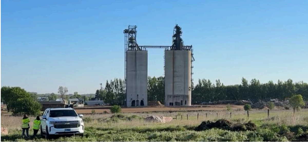
The remaining concrete silos prior to implosion.
