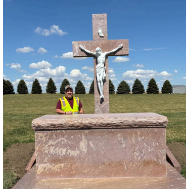
A cemetery cross in Dell Rapids, SD, was recently completed. Made from stone from the Jasper quarry, it was erected by Kevin Moeller, pictured above.
