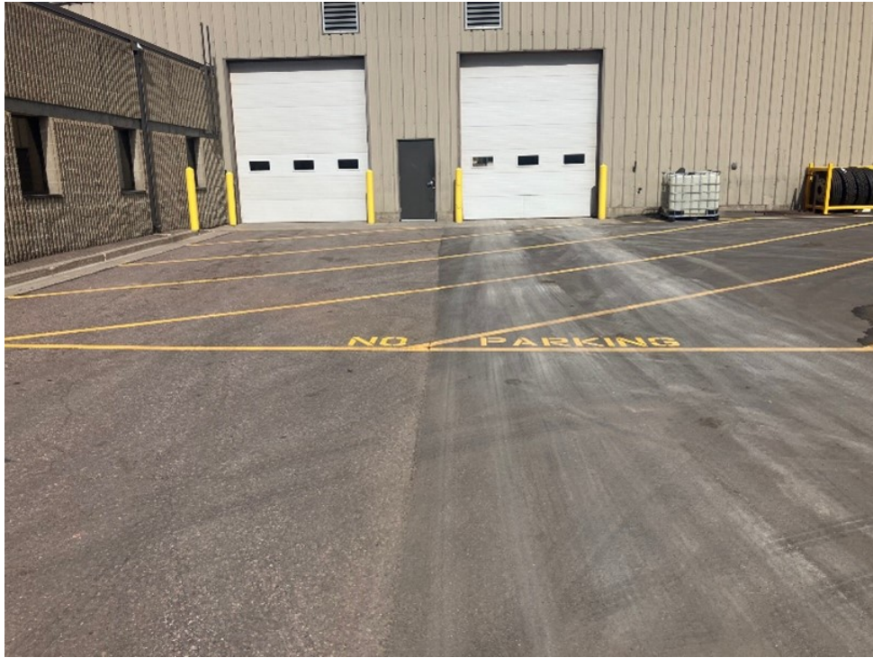
Freshly painted striping outside Myrl & Roy's shop doors.
