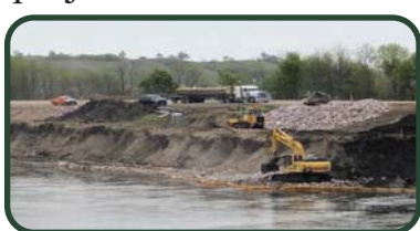
Embankment repairs on the Big Sioux River on IA Hwy 12.
