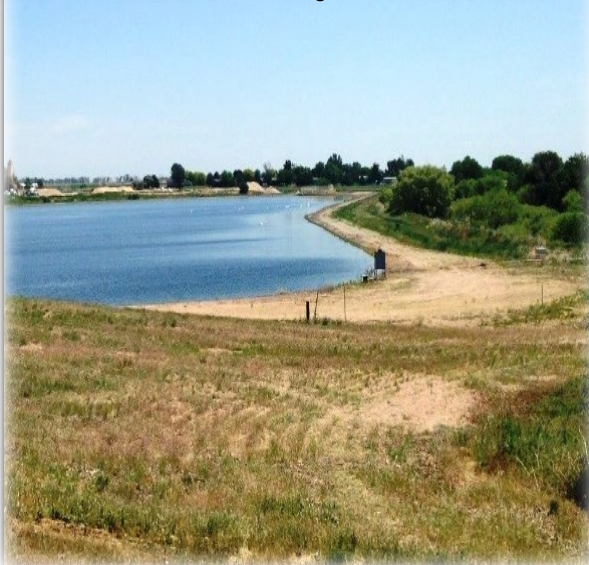
Star - West Lake water storage/access roads
